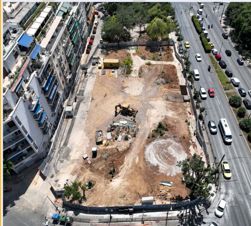
Preparatory work at the EVANGELISMOS TRUMPET Shaft.
