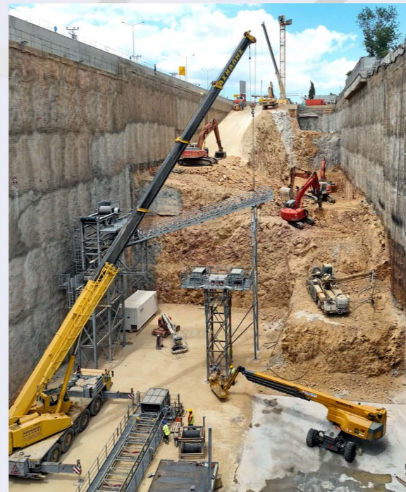
VEIKOU TBM Shaft.
