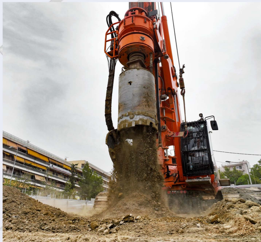
Drilling of piles - GALATSI Station.
