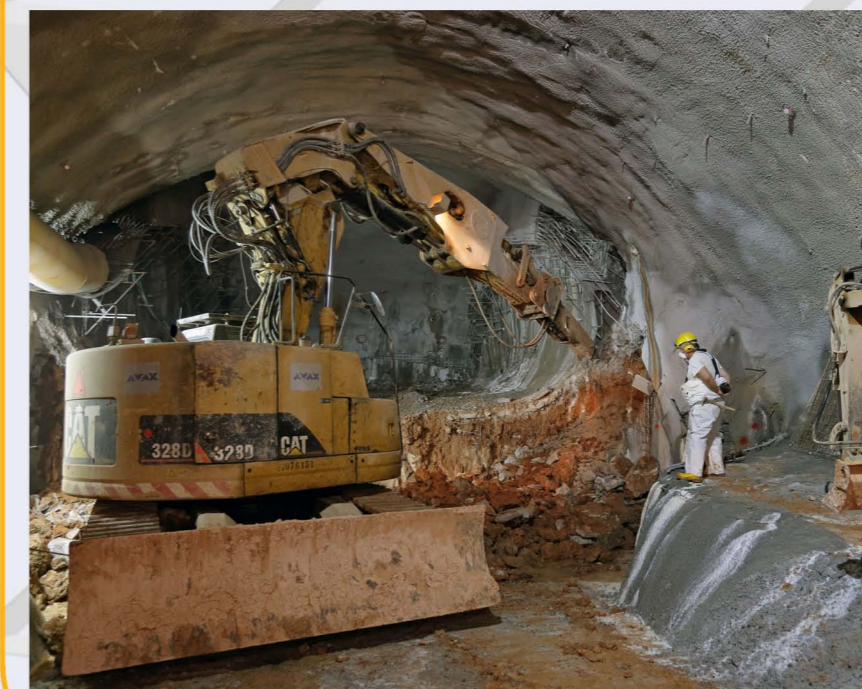
Excavation of access chamber - GNA Shaft.
