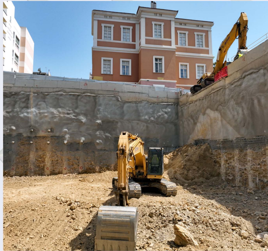
Excavation of the central trench - AKADIMIA Station.
