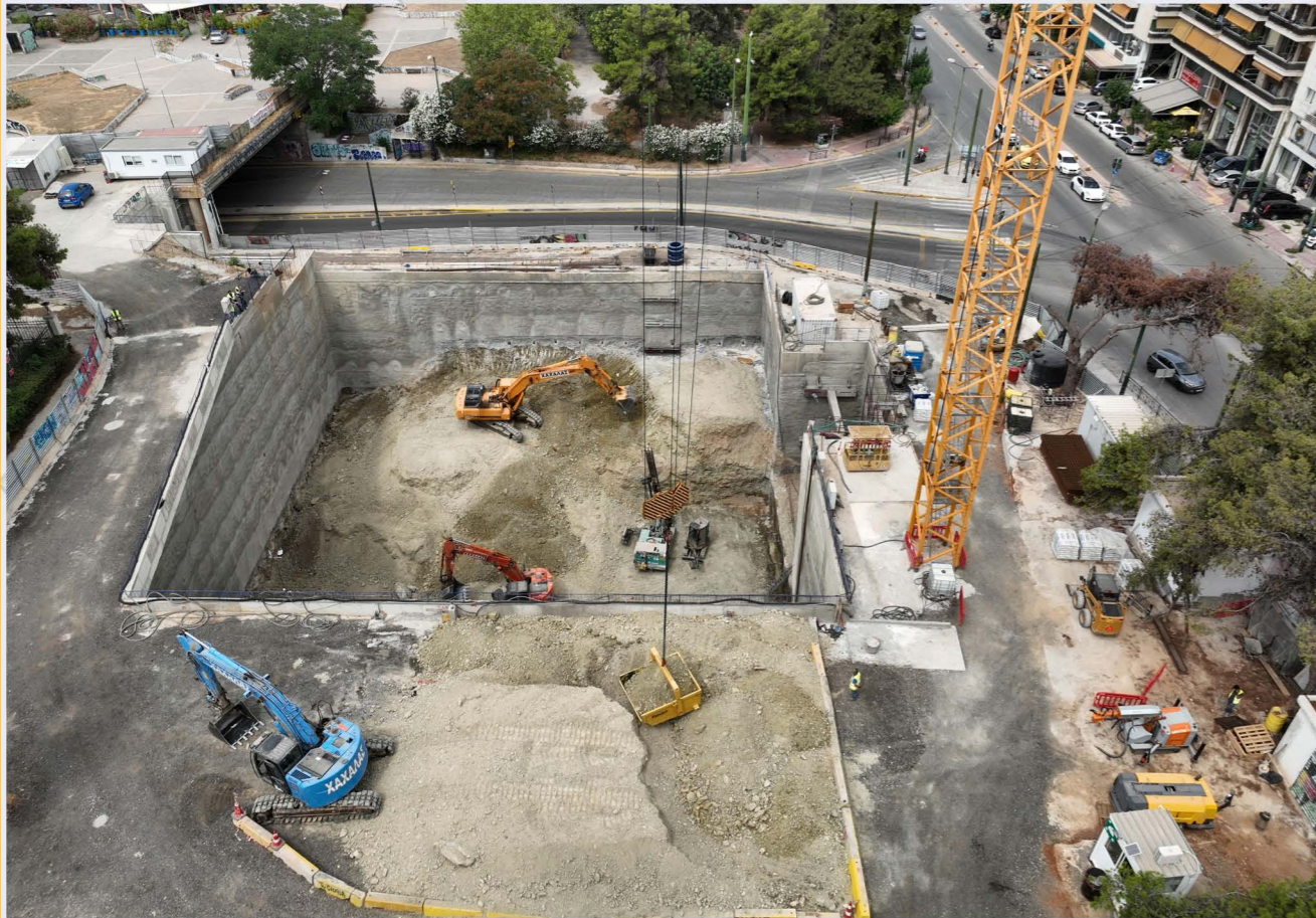
Drilling of anchors and excavation - DIKASTIRIA Station.
