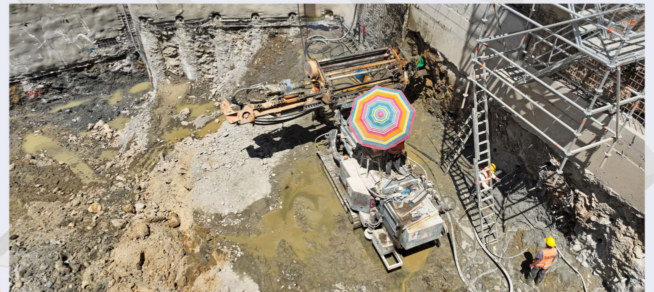
Drilling of anchors - KOLONAKI Station.
