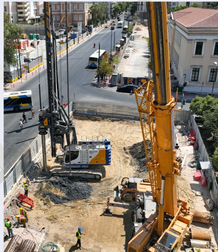
Drilling of piles – VIVLIOTHIKI Shaft.
