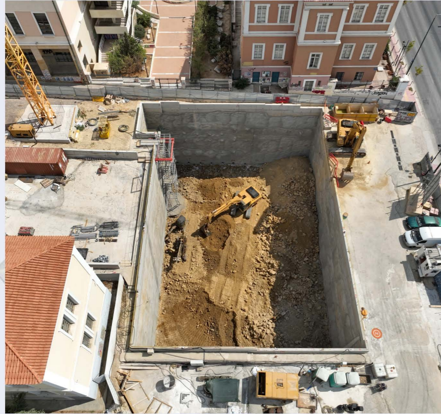
Excavation of the central trench – AKADIMIA Station.
