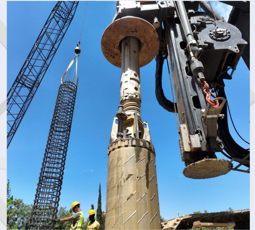
Drilling of piles - EVANGELISMOS TRUMPET Shaft.
