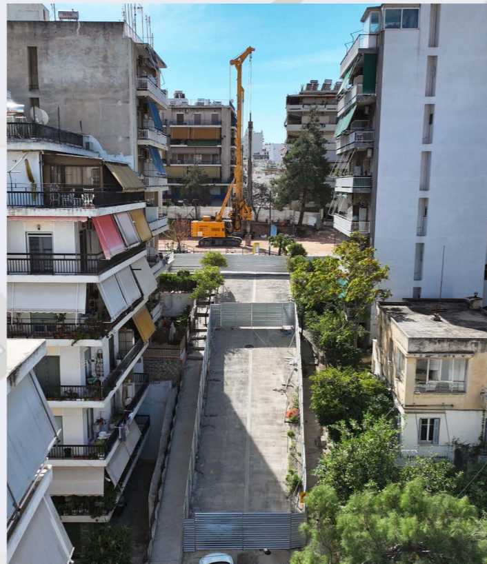
Drilling of piles – ILISSIA Station.
