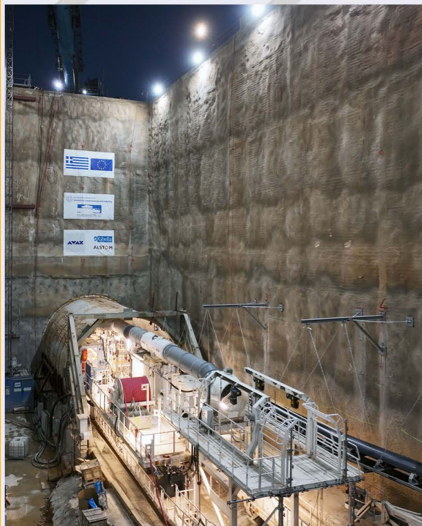
VEIKOU TBM Shaft.
