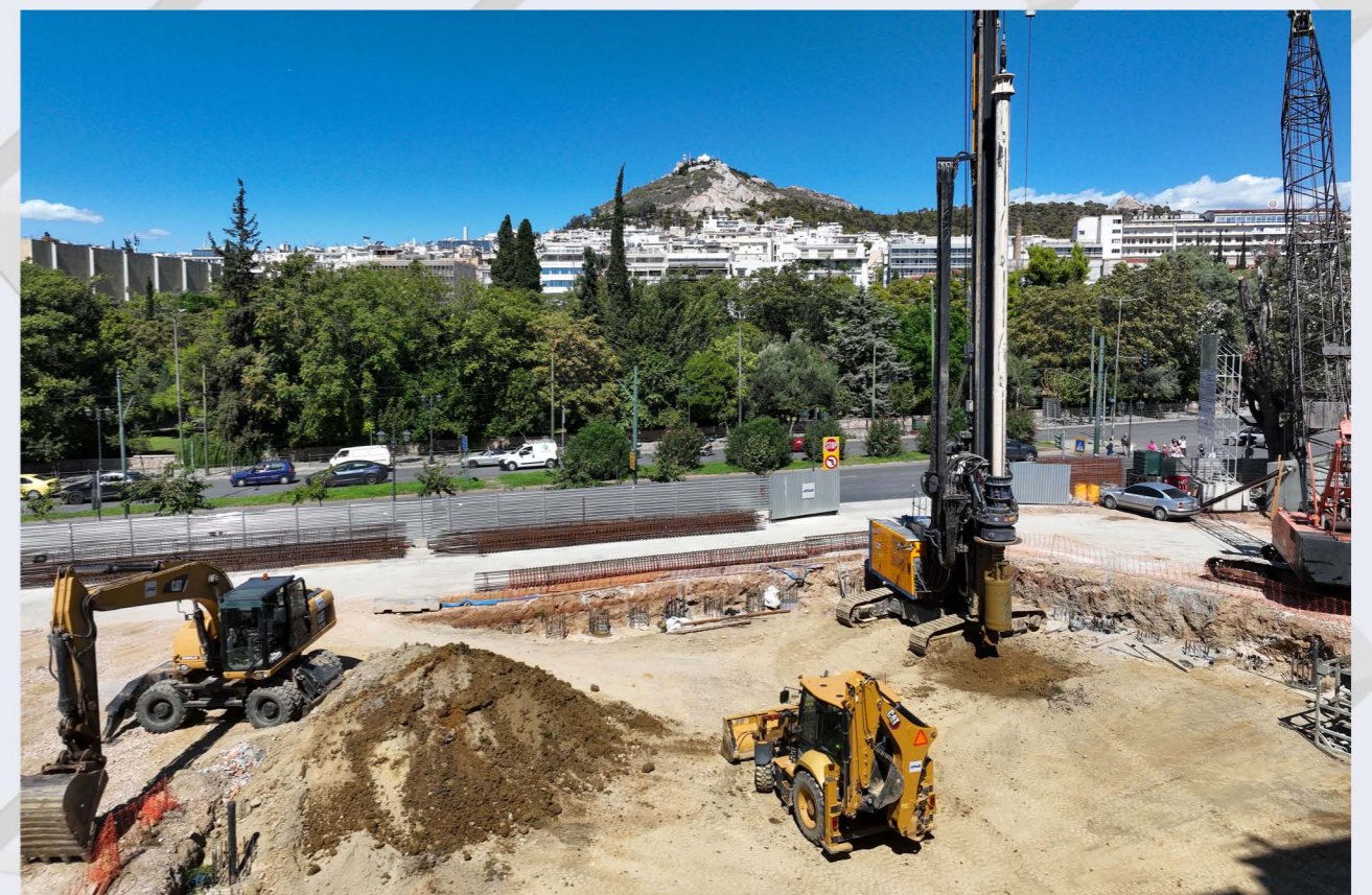
Construction of piles – EVANGELISMOS TRUMPET Shaft.
