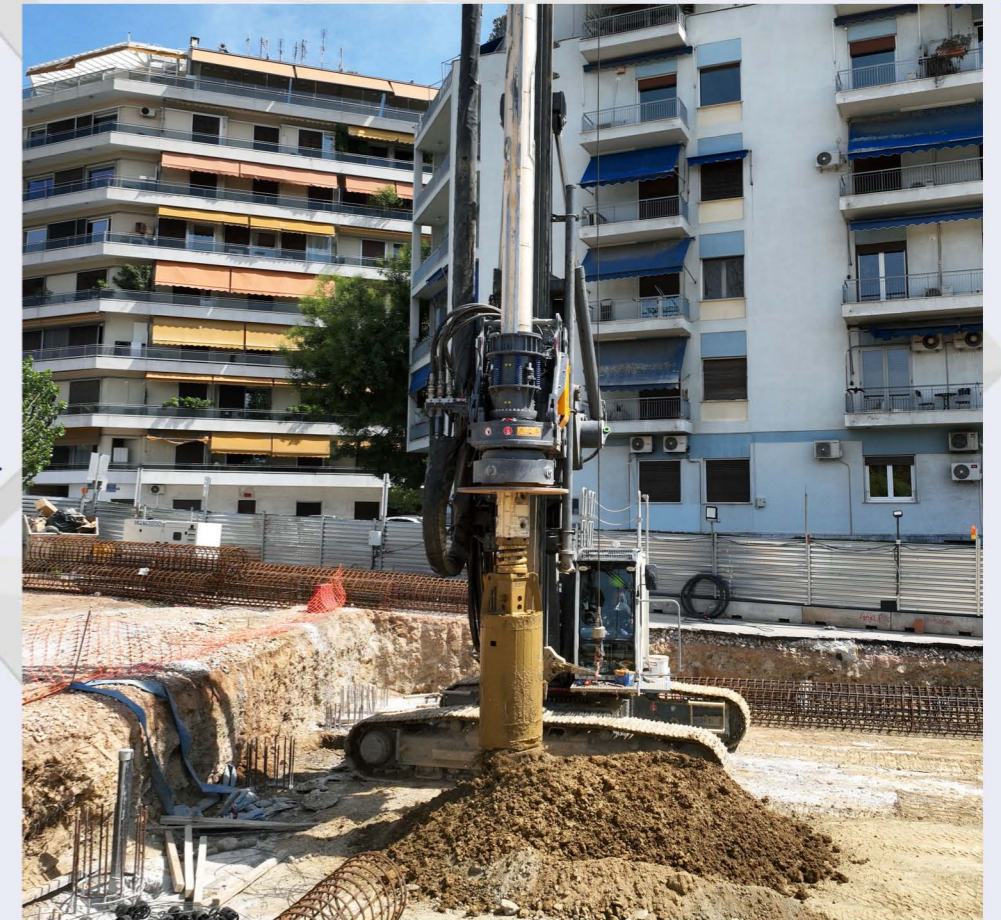
Drilling of piles – EVANGELISMOS TRUMPET Shaft.
