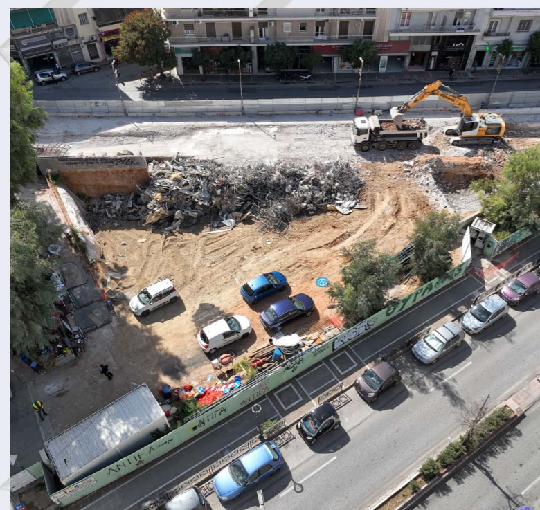
Demolition of building – ZOGRAFOU Station.
