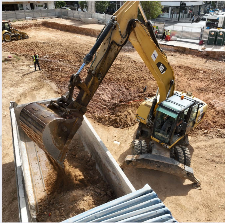
Removal of excavation spoils – KESSARIANI Station.
