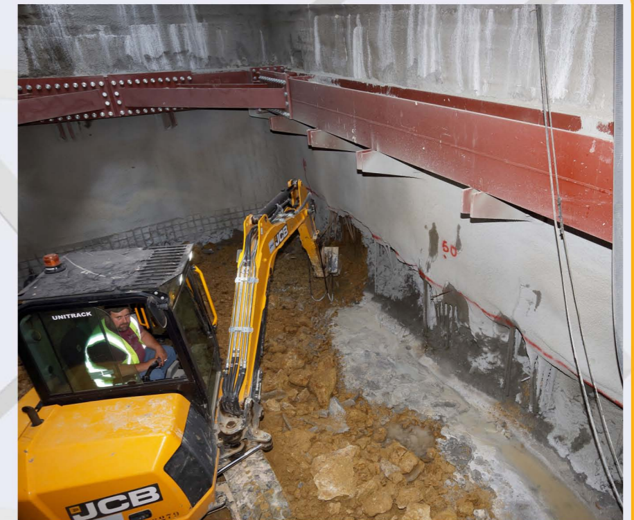
Excavation of the 5th level - EYDAP Shaft.
