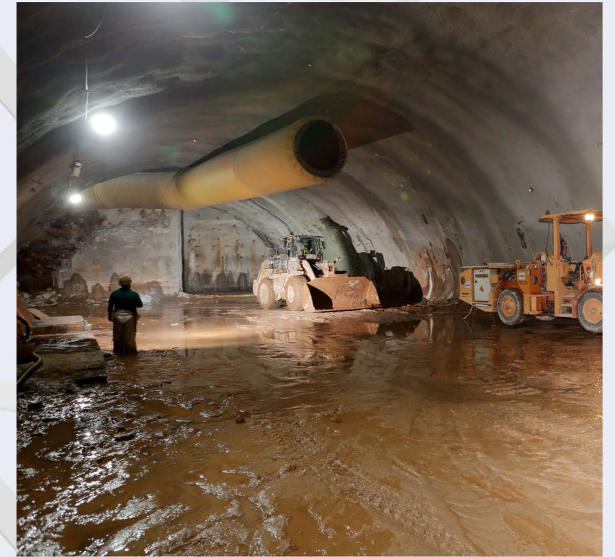
Forestation tunnel – GNA Shaft.
